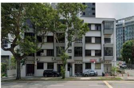
River Valley Apartments
