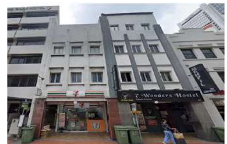
63 & 65 South Bridge Road
